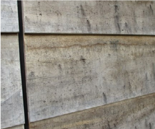
Rough sawn surfaces are more conducive to build-up
