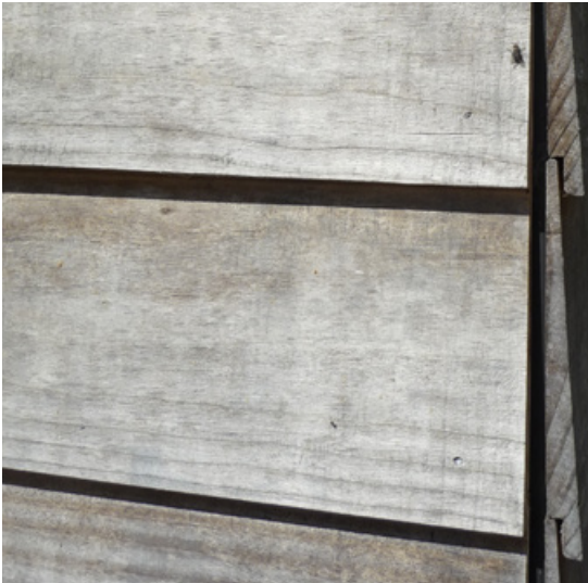
Rough sawn surfaces are more conducive to build-up
