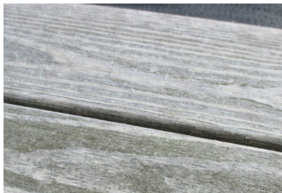
Natural occurring surface fibres on decking.
