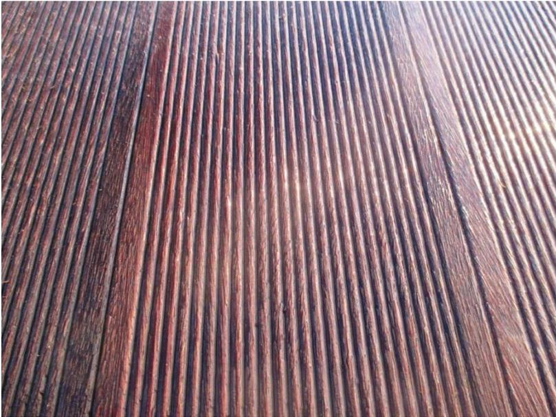
*Figure 4: Bangkirai test deck, originally with 5 mm gaps totally closed up after being exterior exposed.*
